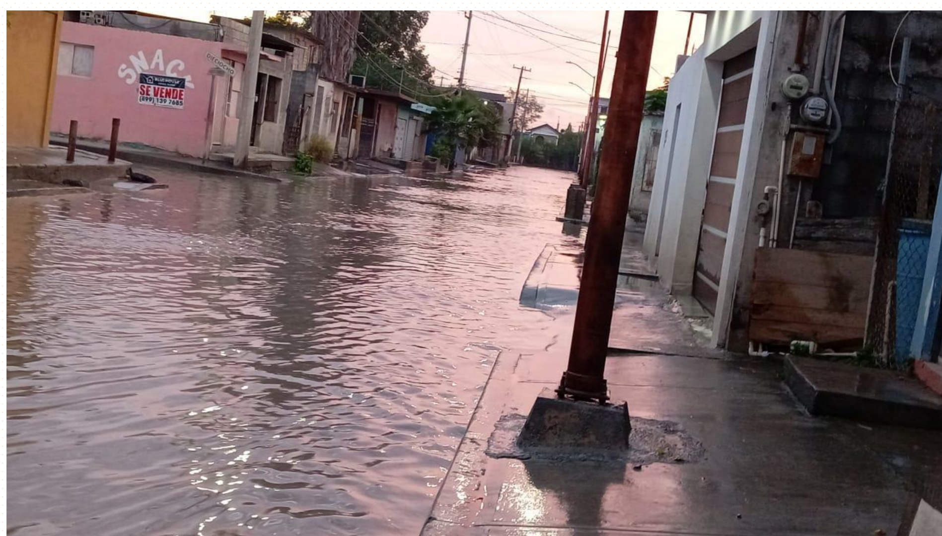
Figure 1.- Representative image of a street flooded due to drainage obstruction caused by contamination.
